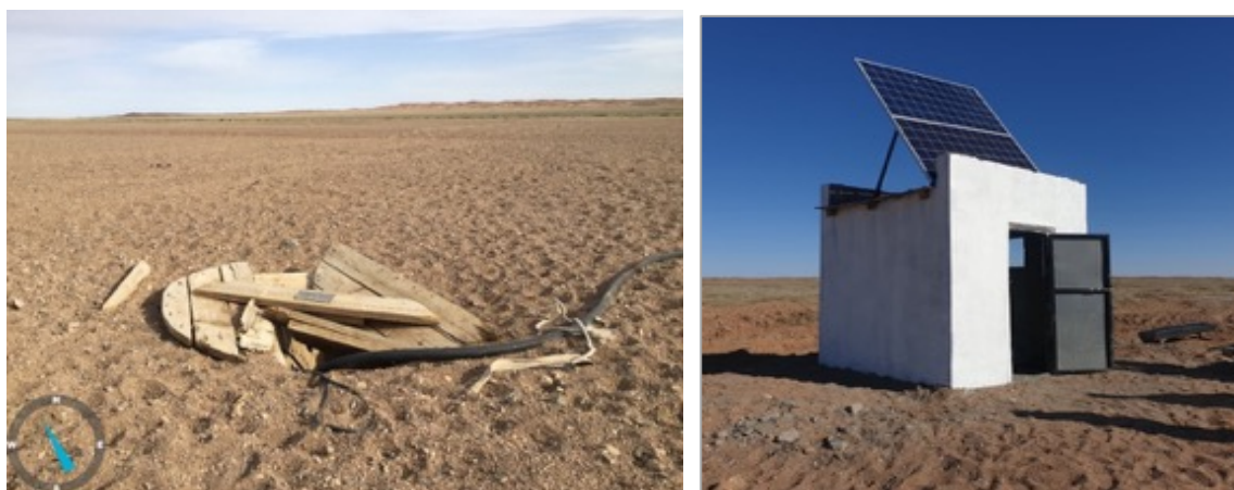
Figure 4-11 Historic Condition of Hand Wells and Improved Version
