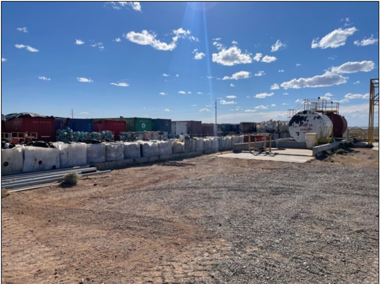
Figure 4-29 Waste Oil Collection Tank with Oily Rag Containment in Background
