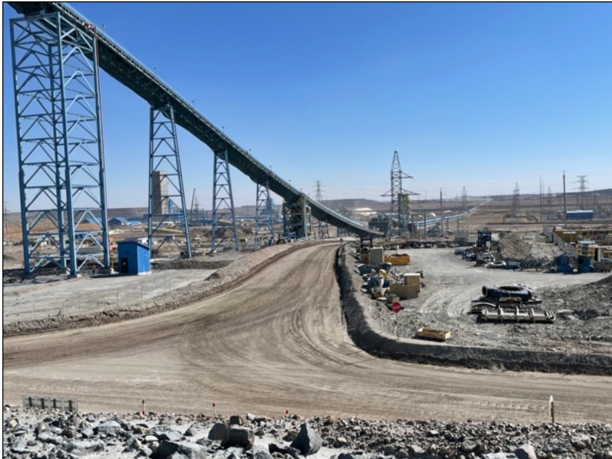
Figure 4-31 Conveyor Delivering Coarse Ore to a Drop Point at COS Facility
