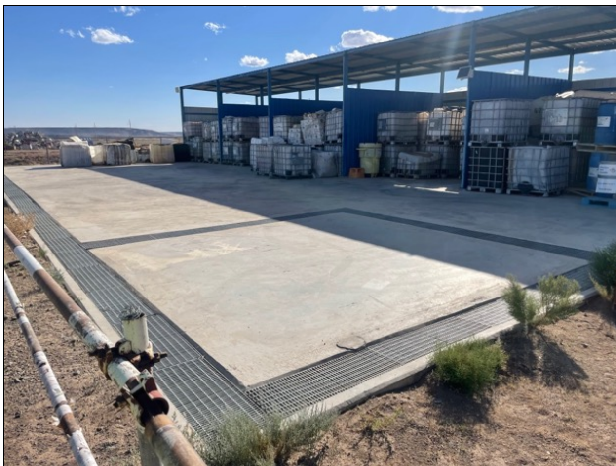
Figure 4-28 Hazardous Waste Storage Area
