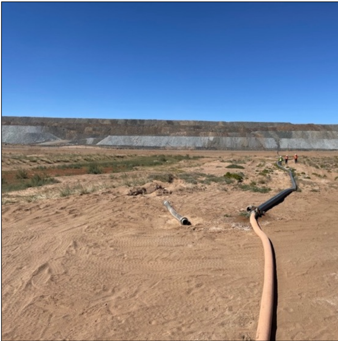
Figure 4-20 Pumping of Collected Waters Back to the TSF
